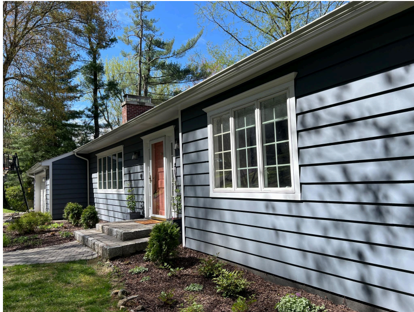
Figure 5. Wall, trim (front)
