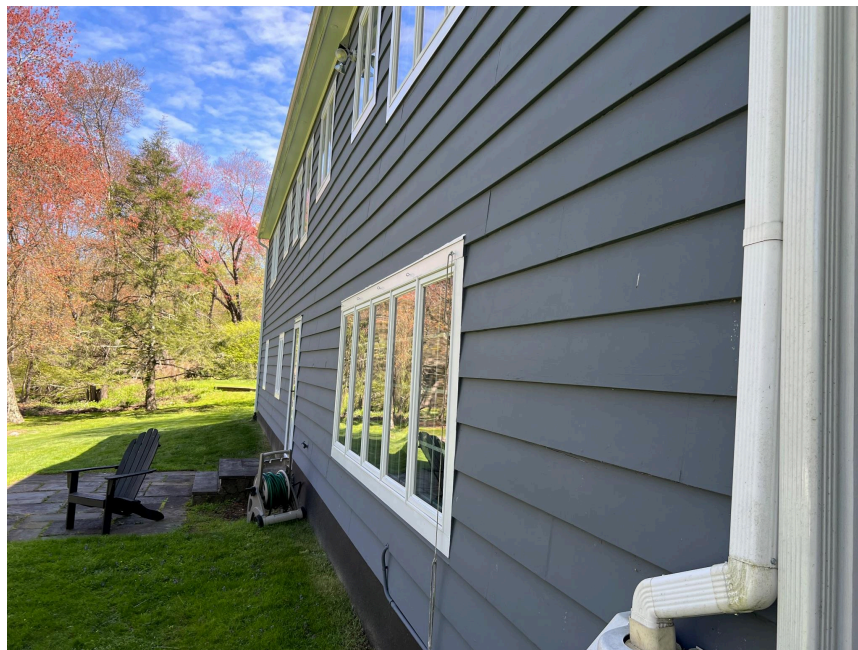
Figure 6. Wall, trim (rear)
